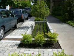
Portland "green street" before and after with rain garden, grate, and permeable bricks to collect and divert stormwater.
