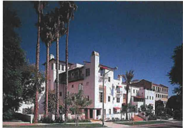
Example of Podium Building
