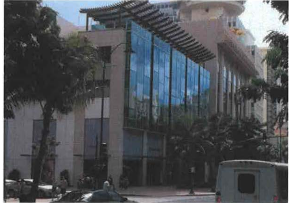
Example of Public Parking Structure
