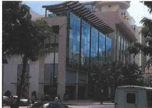
Example of Public Parking Structure
