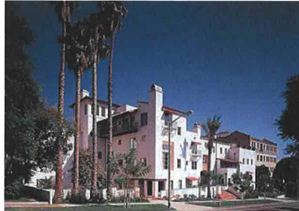
Example of Podium Building
